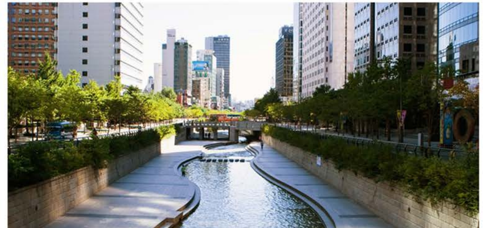
A view of the new canal
